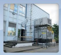
Large scale air cooled projects like cooling this office building are well within our scope. Multiple 25 ton units were stacked to best utilize outdoor space and comfort levels inside were maintained.
