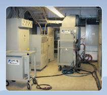
When this electrical vault overheated, the easiest way to power our cooling unit was by utilizing one of our roll-in transformers.
