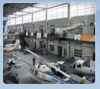
A rather unique opportunity came to Cool Air from this aviation school. The classrooms adjacent to this hangar were sweltering; they were not air conditioned and the learning environment was less than ideal. Positioning these 10 ton air cooled unit on the catwalk allowed for conditioned air to be pumped into the classrooms with the heat rejected to the large air volume of the hangar.
