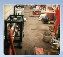
Our 2HP pump was utilized to replace a base building pump that had seized and was two weeks away. The original pump was 600 volt so we added a portable 10kVA transformer to make the installation as simple as possible.
