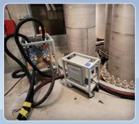
This dual pump set-up allowed for us to move water in two different building circuits. The frame was modified by our technicians to allow for this side-by-side orientation. For over 30 years, Cool Air has customized our equipment based on the requirements of our customers and feedback from our technicians.
