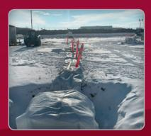
Frozen, snow-covered ground is costly to excavate and can damage equipment. By using this trailered unit, our customer thawed the trench area and coordinated it with their excavation schedule. This predictable thaw-dig-build cycle effectively managed their tight construction timeline, proving both cost-effective and reliable.
