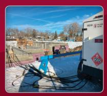
This site's concrete slab was poured the day before cold weather and snow hit. The contractor called for a hydronic ground thaw unit to eliminate the risk from potential freezing. Smart move.
