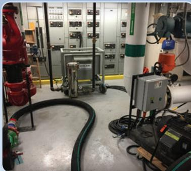
The primary and back-up chilled water pumps for this 20-storey office tower failed within one week of each other. The quick succession of failures meant the HVAC contractor didn't have the primary pump replaced in time, and once the back-up pump failed, the building was left without any cooling circulation. We got an urgent call and had the solution in place and operational by the next morning.
