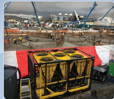
We provided a chiller package to manage the vast amount of heat generated during the curing process of this large concrete pour. Our pump circulated water through almost 8km of 1" PEX tubing that was attached to the reinforcing steel of this raft slab. We managed the project on a daily basis until the internal heat dissipated and the design conditions deep inside the slab were achieved.
