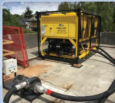
This chiller supplied temporary cooling to the main tower at Vancouver City Hall. The static pressure in the main lines was more than the on-board chiller pump could overcome. By adding this 30 HP pump into the circuit, we were able to move the cooling fluid throughout the building.
